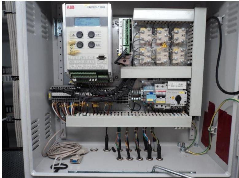
Slika 2.4: Automatski regulator napona generatora (eng.: *Automatic Voltage Regulator, AVR*)
