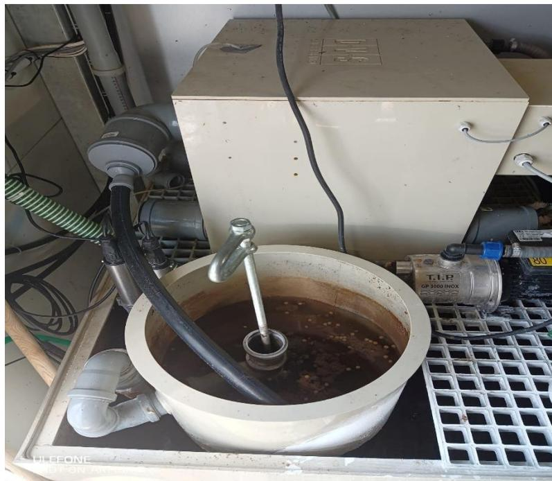
Figure 4. Mechanical filter and vortex where most of the waste is collected from the RAS (source: M. Prečanica).
