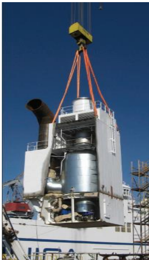
Slika 13: ukrcaj scrubber pred instalaciju na brod pomoću lučkih dizalica (izvor: Alfa Laval: Understanding exhaust gas treatment systems , 2012., Retrofitting of a closed loop scrubber with baypass )
